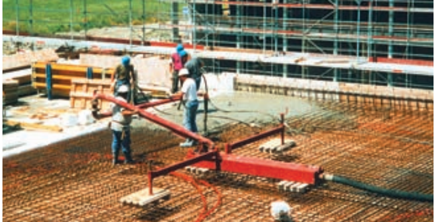
The rotary distributor RV 7: Weight without ballast 610 kg · ballast 280 kg
