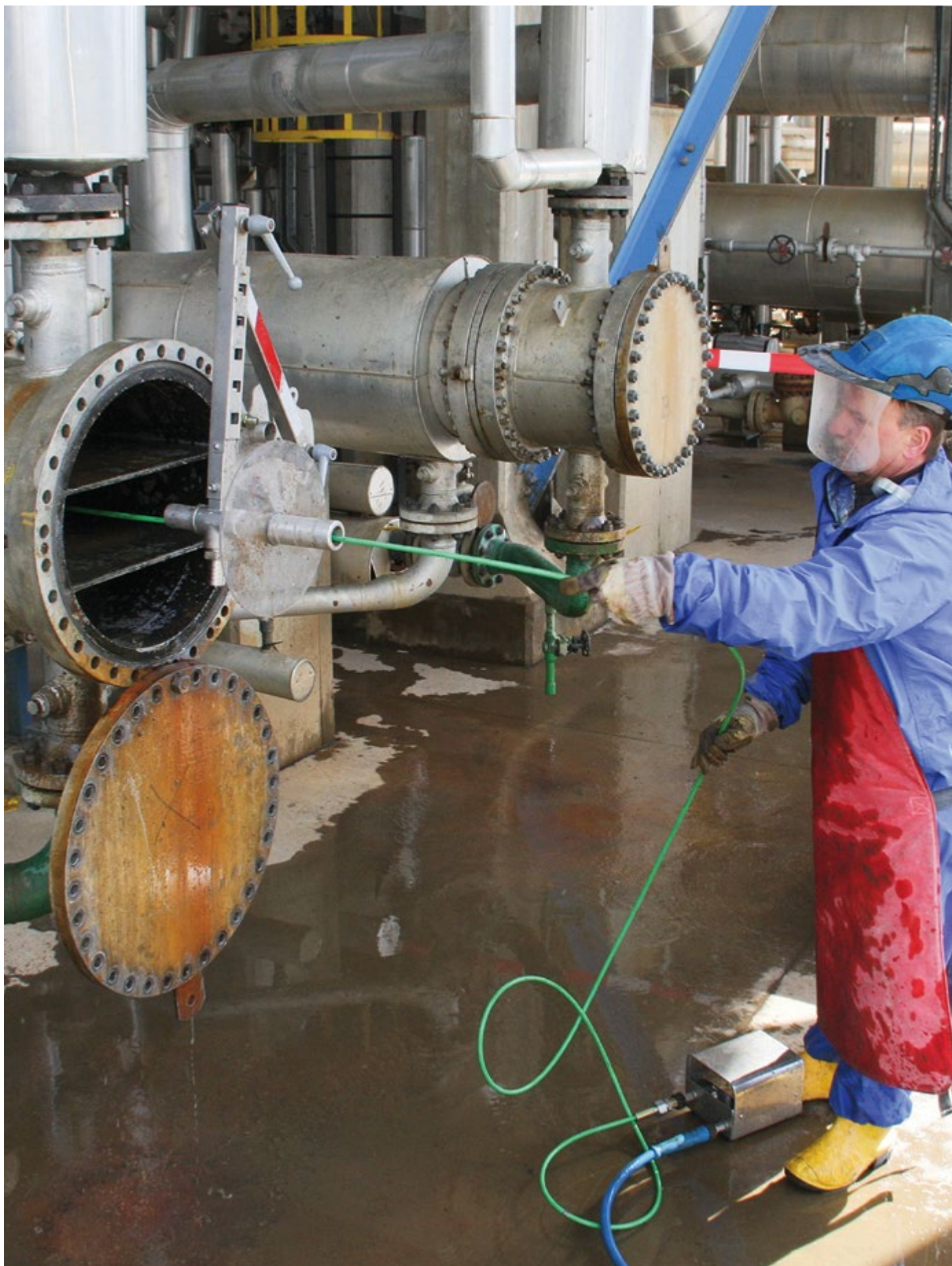
Cleaning heat exchangers
