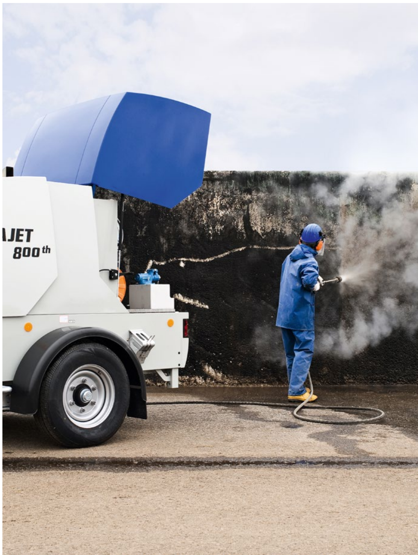
Restoring a bunker silo
