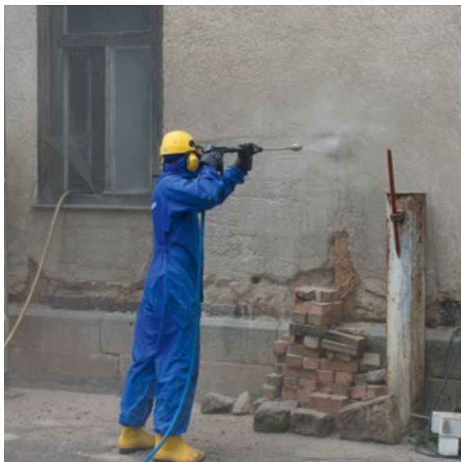
Renovating a facade
