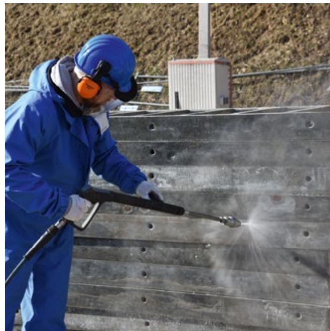
Cleaning shuttering
